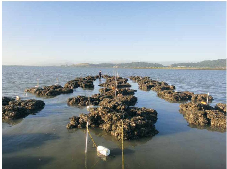
Constructed reefs with Pacific shell bags provide hard substrate in SF Bay.
